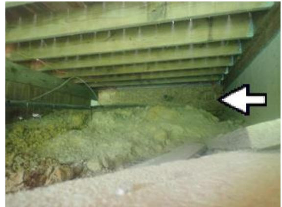
Bare OSB Board under Porch
