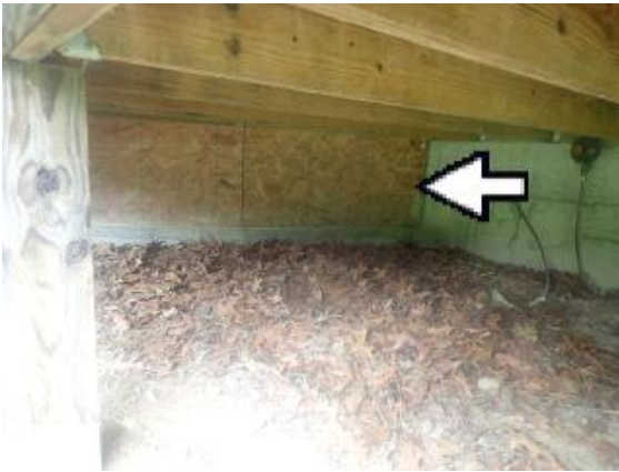
Bare OSB Board under Porch
