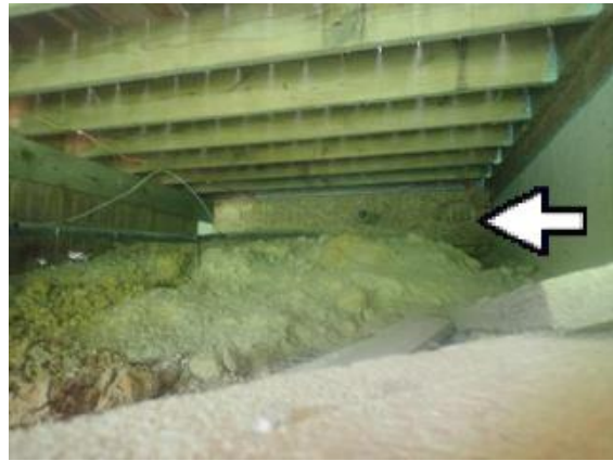
Bare OSB Board under Porch
