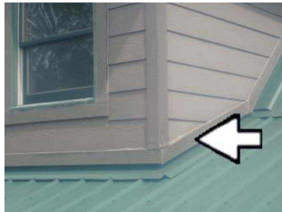
Bare OSB Board under Porch
