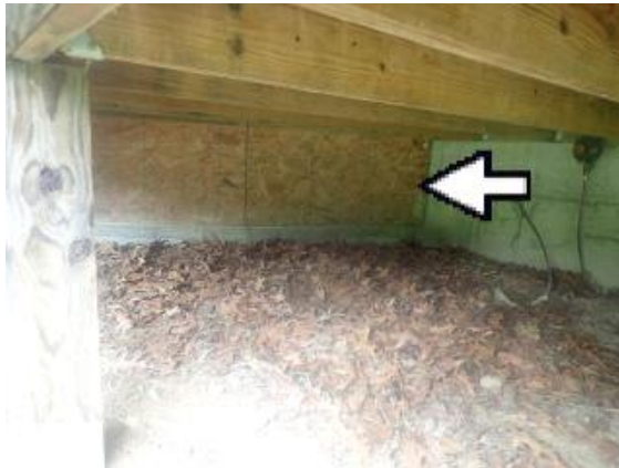
Bare OSB Board under Porch
